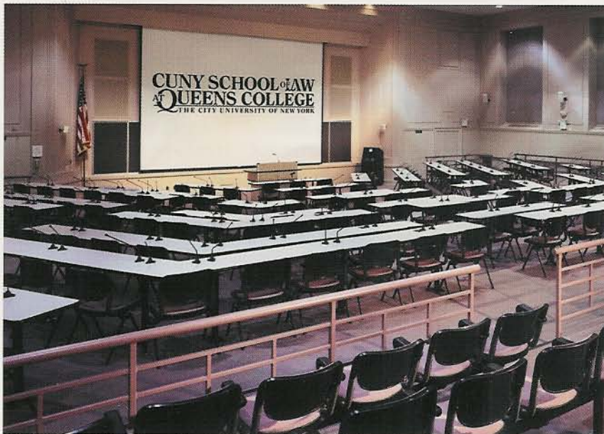
▲ The City University of New York Law School at Queens College in Flushing, NY has upgraded the sound system in the school's main lecture hall. A total of 159 Audio-Technica Engineered Sound ES905/H rigid-pipe microphones (below, right) were installed in the hall.
